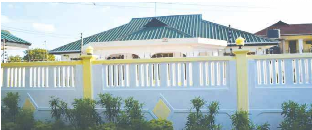
THRDC well protected office
